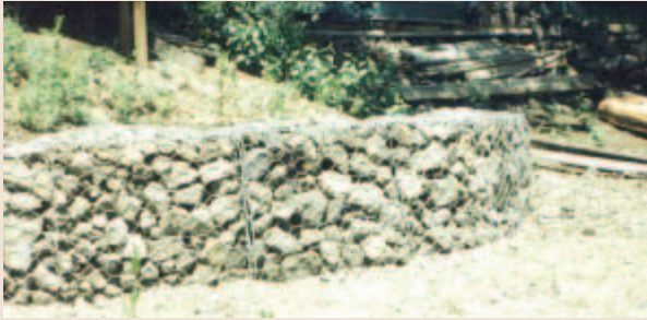
A close up of gabion wall baskets filled with small to medium size rocks; they are typically placed on moderate slopes with minimal to moderate wave action.
